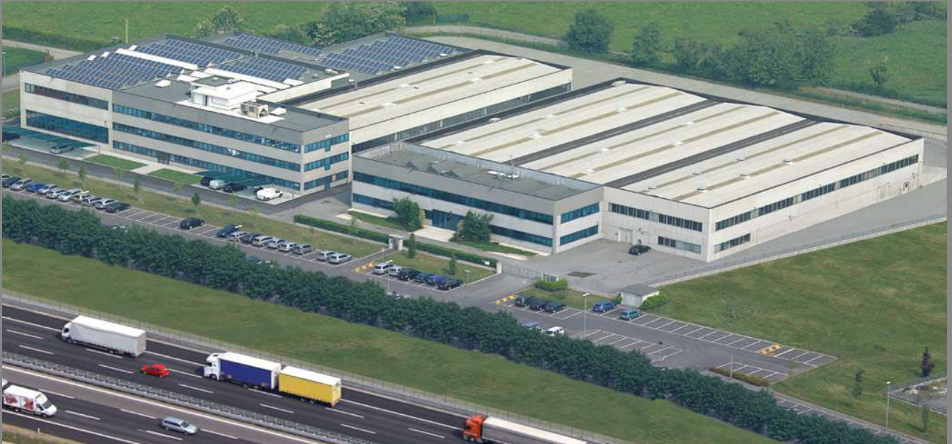
Maico Italia SpA headquarters in Lonato del Garda (Brescia), Italy
